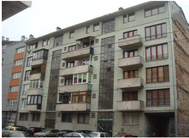
Slika 1. Analizirana zgrada u Sarajevu, Bosna i Hercegovina (fotografisao autor) Figure 1. Analyzed building in Sarajevo, Bosnia and Herzegovina (authors' photo)
